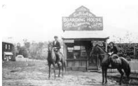
E. & H. Law's boarding house, corner of Farrell Street and Stevens Street, Yandina, 1920s, originally owned by Mrs Murray (1896-ca 1903). It was used as a private residence for some years until it was acquired by the Law family. The building was demolished in 1988.
