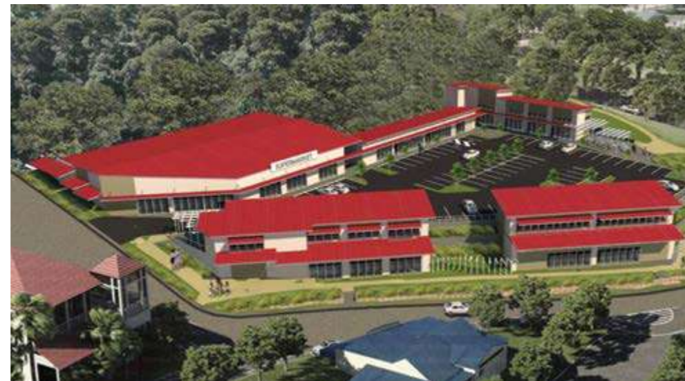
The shopping centre is planned for Main, Hill and Church streets in Palmwoods, opposite the Palmwoods Hotel and train station.
