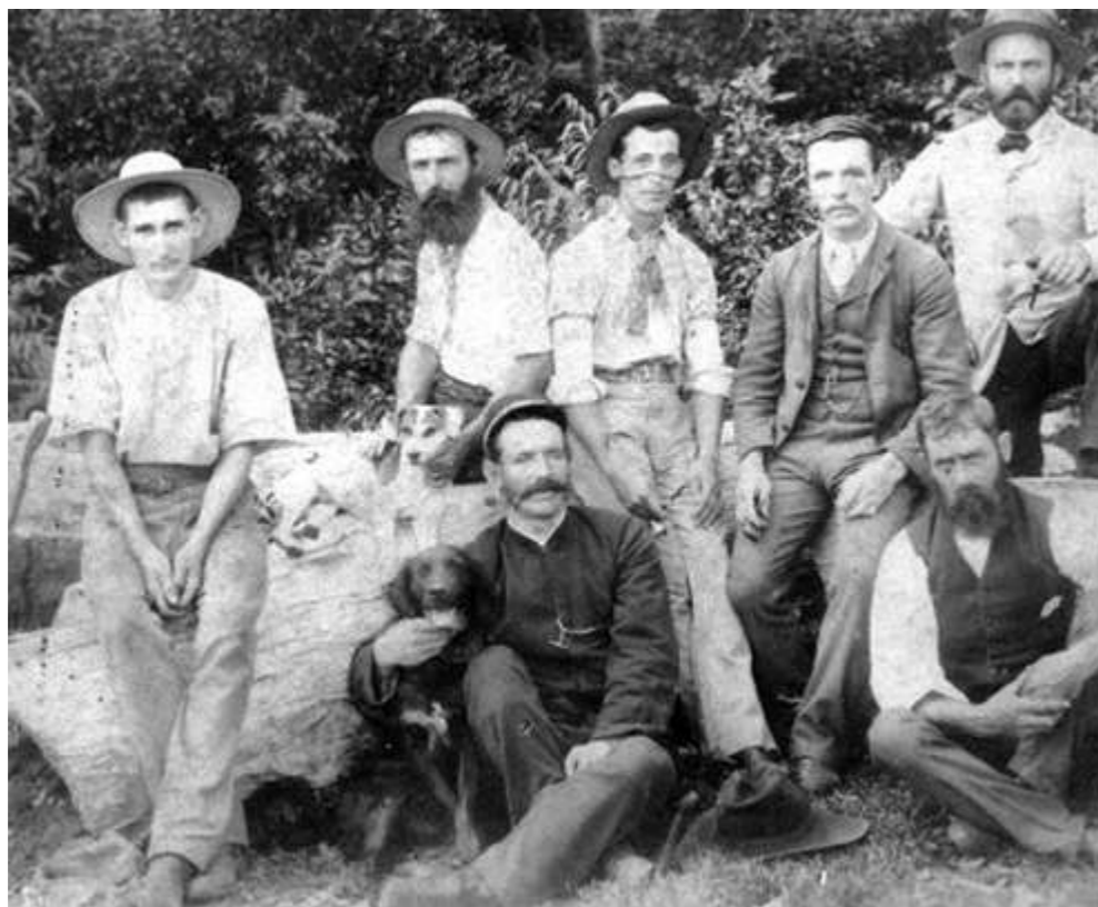
Men pictured during the clearing of land for the construction of the Excelsior Hall, ca 1900. Pictured: Alex G. Low (far left), John Gustave Sommer, far right, his brother Richard Bernard Erwin Sommer, in dark suit seated on log, Mr Mitchell, Yandina Station Master (seated in front with dog).
