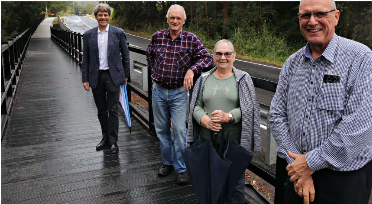
Cr David Law inspects the Zealey Road boardwalk with newest Sanctuary Park Retirement Community resident Bill Turner, the community's first resident Gwen Rose and Manager Russell Elms.
