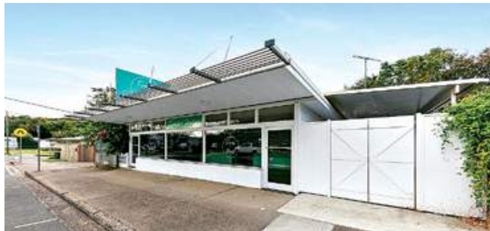
There are huge glass windows at the north-facing front inviting in abundant natural light.
