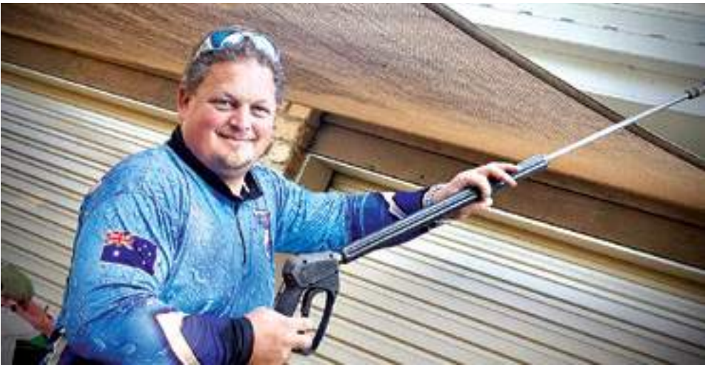
Jon McCabe, owner of Water Attack Pressure Washing , has blasted clean several prominent facades in town.
