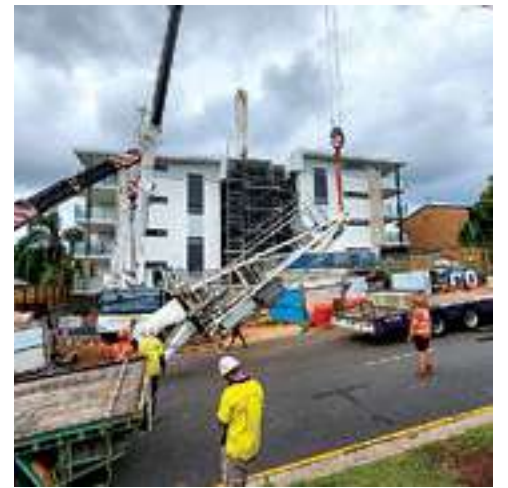
Cranes being demolished in January.
