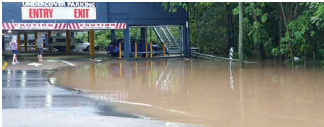
Within an hour, the water was lapping at the edge of the carpark under Superheap Auto in Nambour. Photo: Dale Myers
