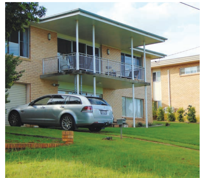
The planned carport would be partially screened by trees on the neighbour's property.
